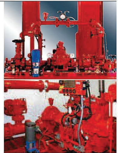
Pictured at top: Packaged Fire Pump System.
